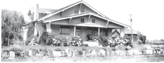
House in Elgin built by Laurose's parents, 1921, (all architectural features are Craftsman style, retained as of 2003)
